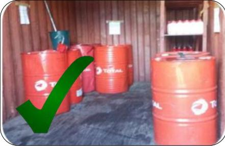
Disused fuel tanks awaiting recycling should be stored at a safe distance from potentially flammable materials and spark sources and over a protected hard surface.
