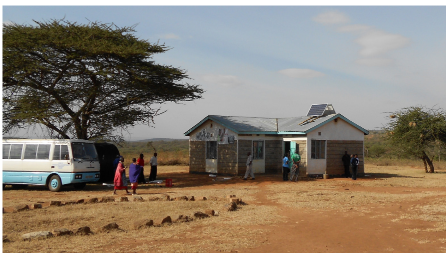
Solar panels on the roof of Pelewa dispensary, Kenya. Photo: Catherine Silali.
