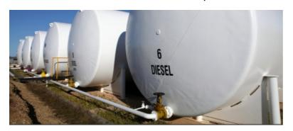
Linked tanks enable storage planners to "right size" their storage needs, using as much or as little storage as required. Linked tanks can even be used to push fuel between reserves with specialized equipment and pumps.
